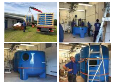
On site assembling
